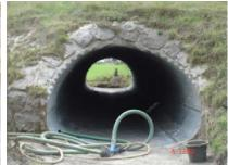
Ready for blasting and coating the culvert steel.
