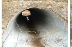
Brushing out the sand and soil before blasting.
