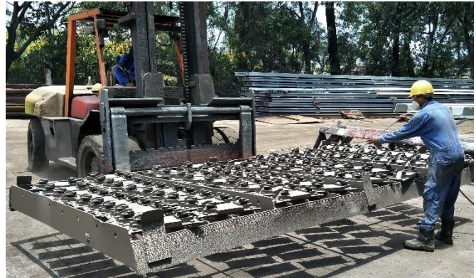
Dedusting of the baseplates
