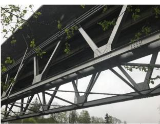
These photos are from May 2017, after 15 years of exposure. The system is still intact without any sign of breakdown or failures. Even in complicated areas such as around bolts, nuts and rivets there are no failures. The system is believed to protect the steel structure for many more years to come.
