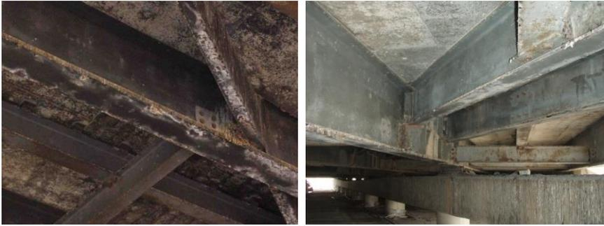
These pictures clearly indicate the high degree of corrosion before refurbishment with the **ZINGA** system.
